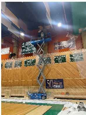
Scissor Lift & Floor Protection
