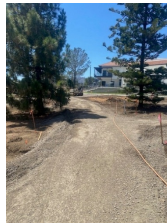
Walkway Fine Grading
