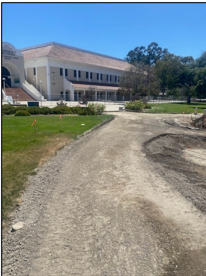
Grading & Compaction
