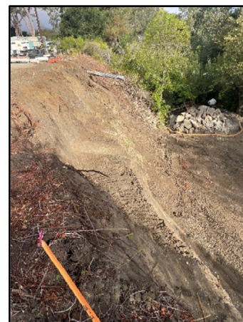
Downstream Bench Slope
