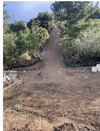
Surveyed Work Pad
