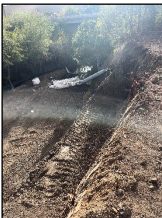
Upstream Bench Slope
