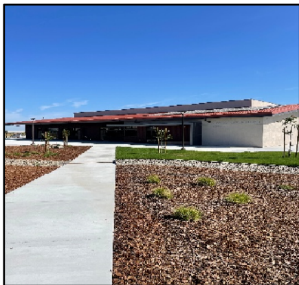
South Facing Facade
