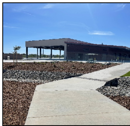
West Facing Facade
