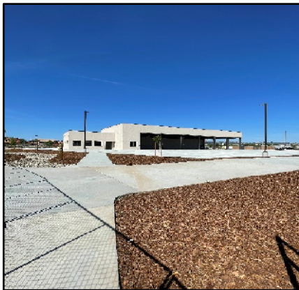
North Facing Facade
