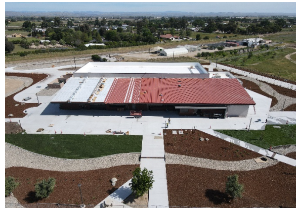
NCC Instructional Building from Above
