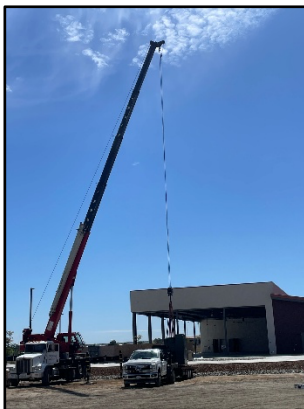
Temp Transformer Change Out
