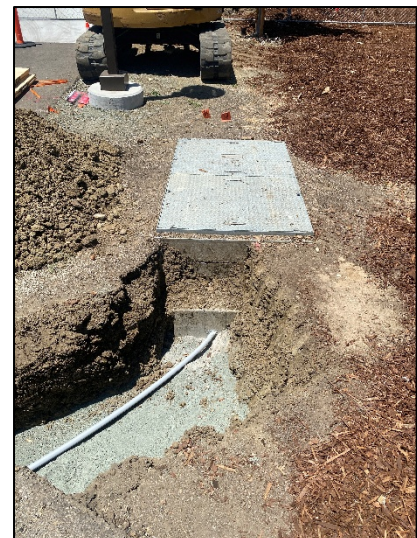
Electrical Install Cont.
