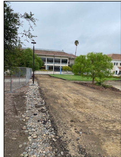
Asphalt Pathway Demolition
