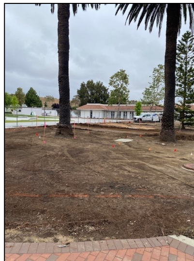
Site Survey Continued
