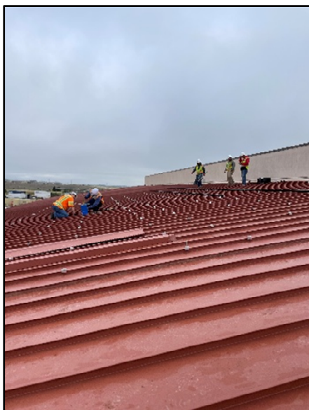
Solar Array Load Testing
