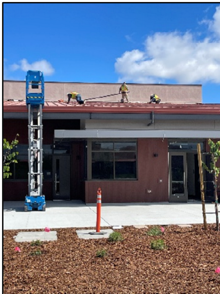
Solar Array Racking Installation
