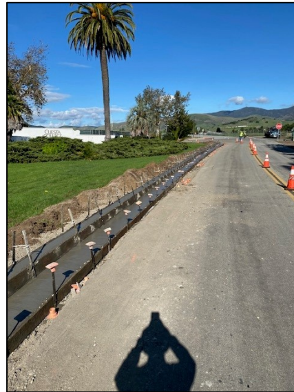
New Curb & Gutter
