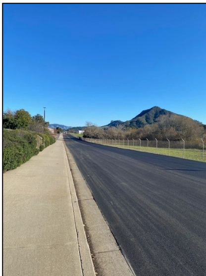
Asphalt Overlay
