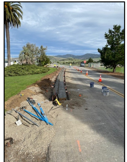
New Curb & Gutter
