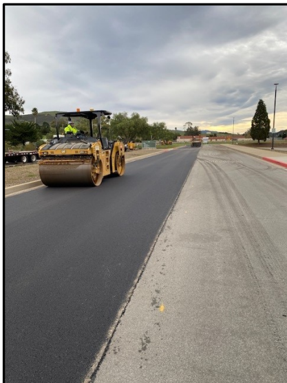
Hot Mix Asphalt Overlay
