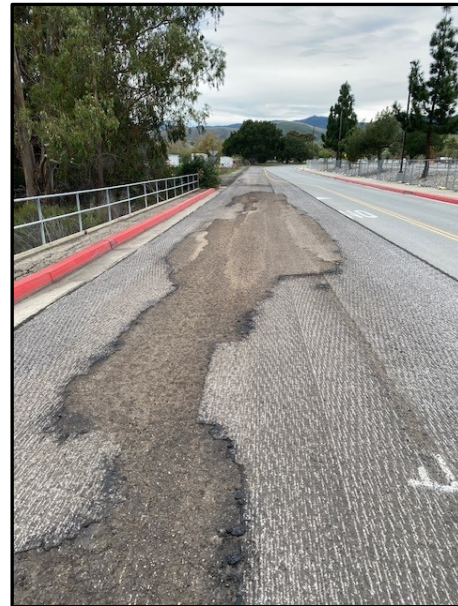
Asphalt Grinding
