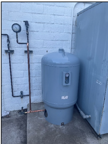
Boiler System Expansion Tank
