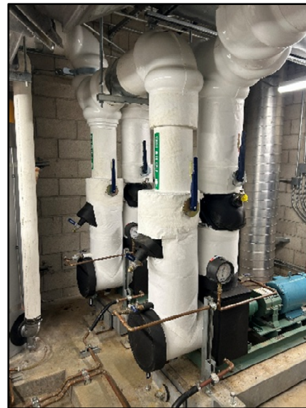
Chiller Pump Pipe Insulation
