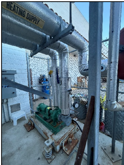
Boiler Pump Pipe Insulation
