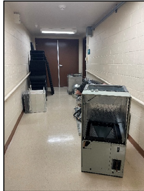
Evaporator Replacement
