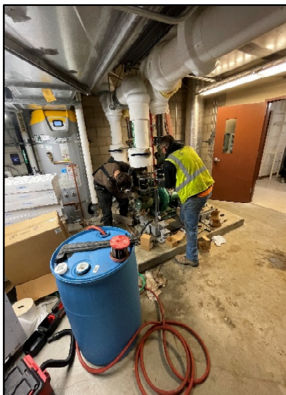
Chiller Pump Replacement
