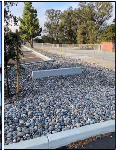
Exterior Signage Bases
