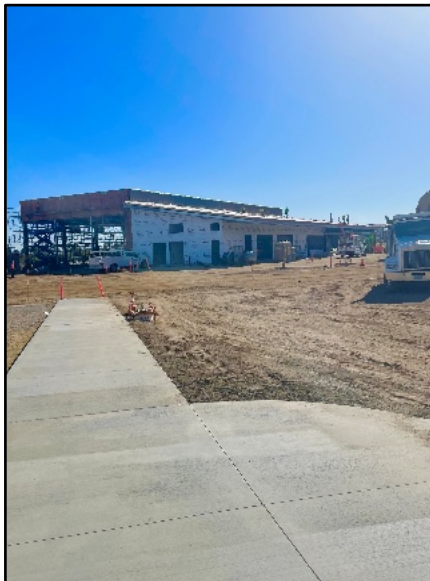
Building Paper Installation
