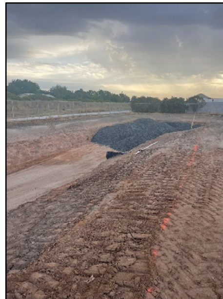
South Retention Pond
