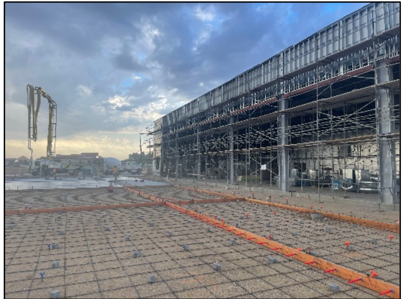
Building Open Area Apron
