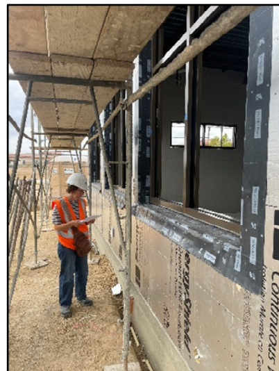
Window Flashing Mockup
