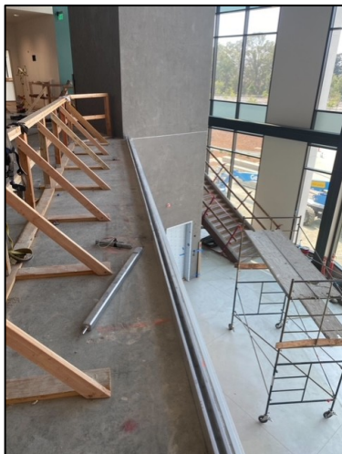
Structural Glass Guardrail
