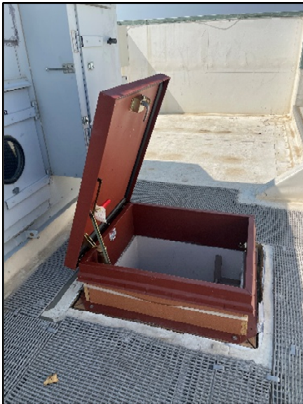
New Roof Hatch
