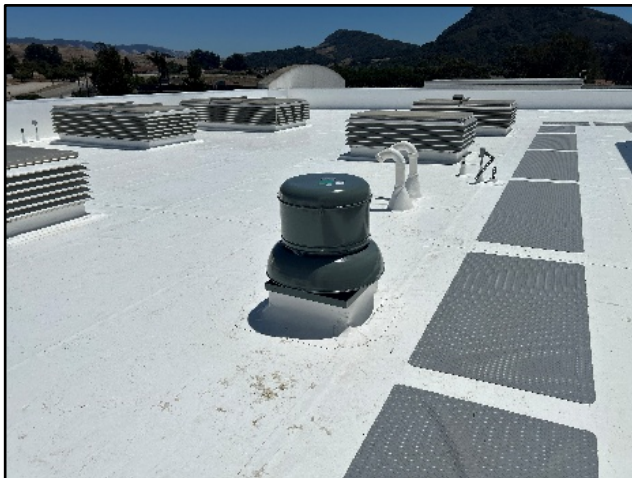
New Exhaust Fan and Walkway
