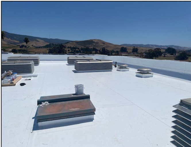
Roof Membrane Replaced
