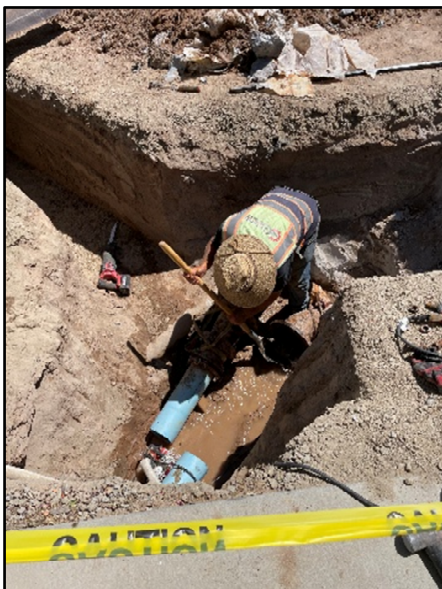
Fire Hydrant Connection
