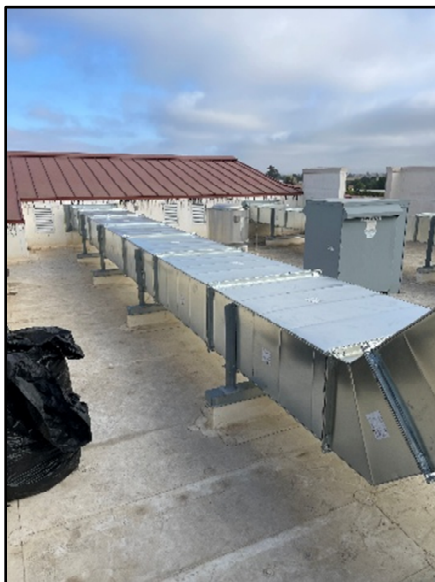
New Duct Material Installed
