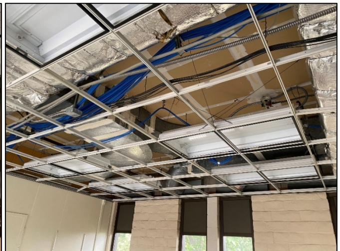
Acoustical Tiles Removed
