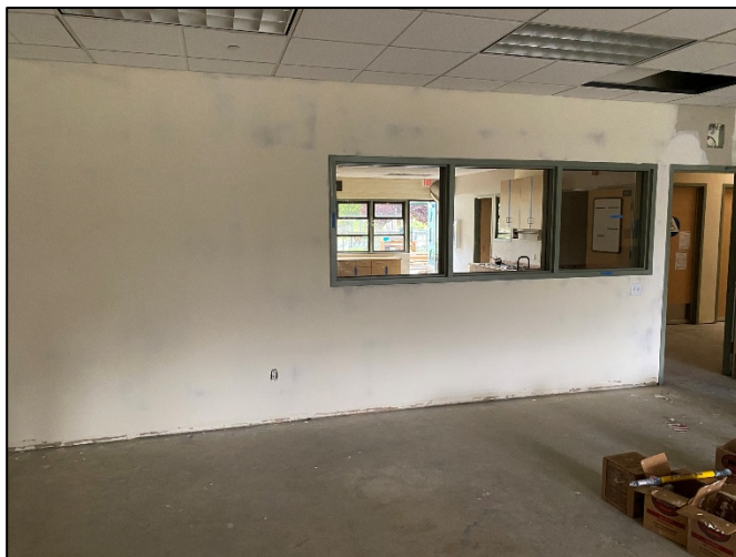
Drywall Patching Complete
