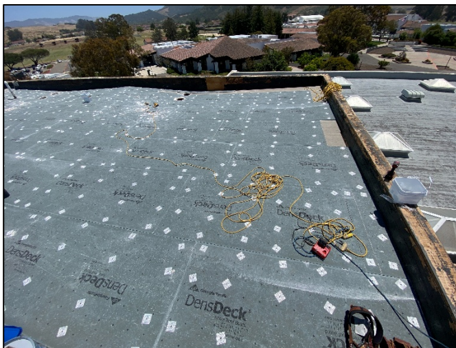
Roof Board Install
