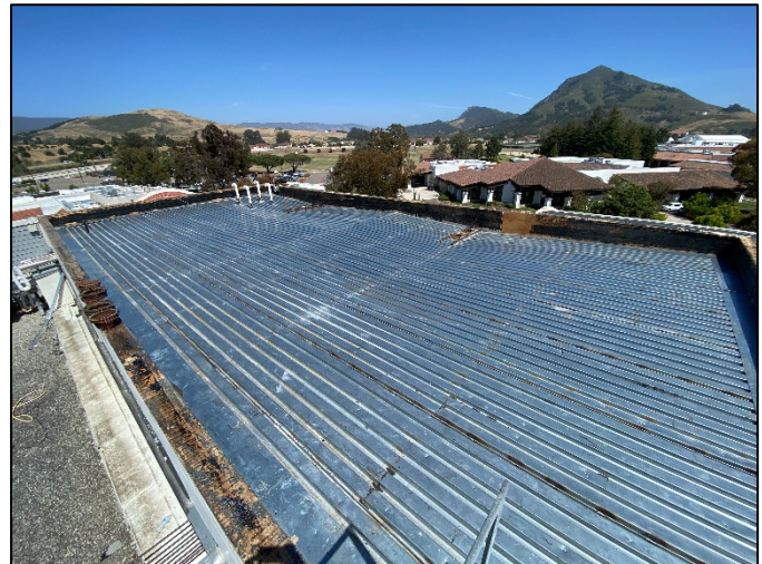
Existing Roof Removal
