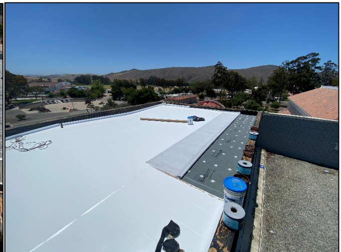
Weather Membrane Install
