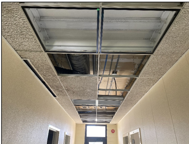
Acoustical Ceiling Removed
