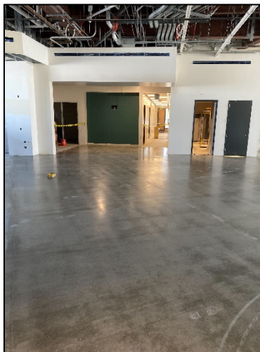
Concrete Polishing
