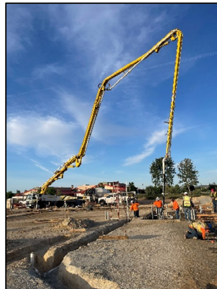
Concrete Pumping
