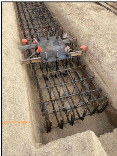
Grade Beam Reinforcement
