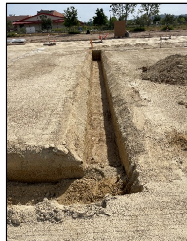
Under-slab Plumbing
