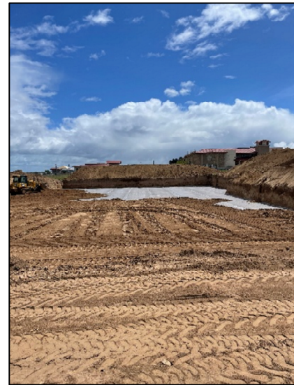
Backfill & Compaction
