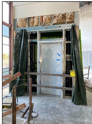
Elevator Install
