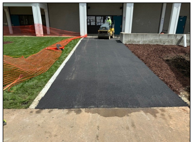
Asphalt Install
