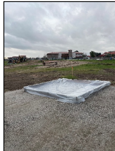
Concrete Cleanout
