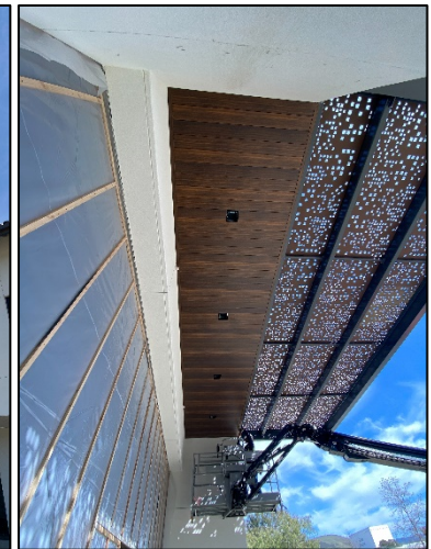
Metal Panel Installation
