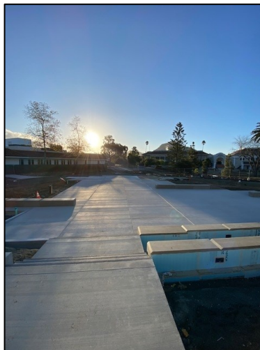
Concrete at Amphitheater
