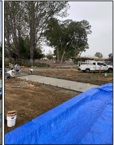
Concrete at Amphitheater
