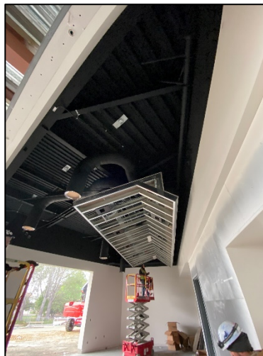
Framing at Cafe
