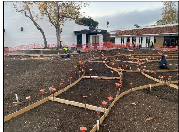
Concrete Formwork
