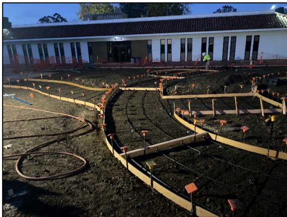
Concrete Formwork
