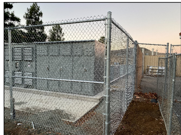
Perimeter Fence Installed
