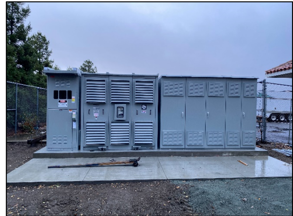
Electrical Equipment Installation
