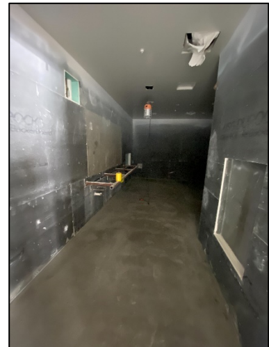
Mortar Beds - Restrooms
