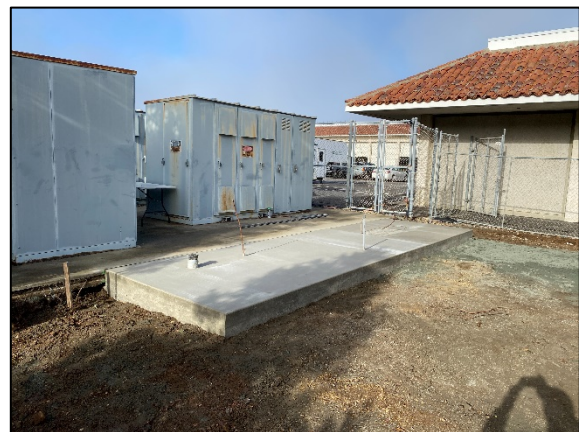
Concrete Slab Poured
