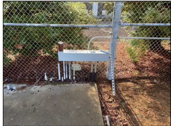
Electrical Wiring Installed
