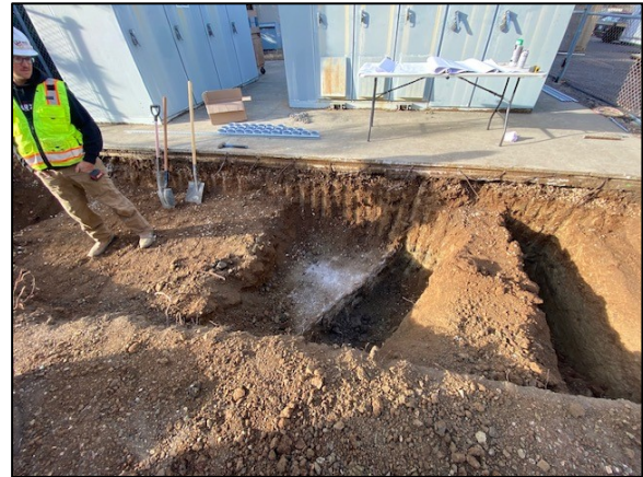
Demolition and Excavation
