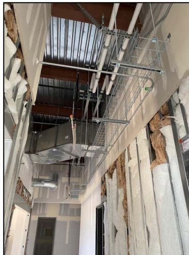
Cable Tray – 1 st Floor
