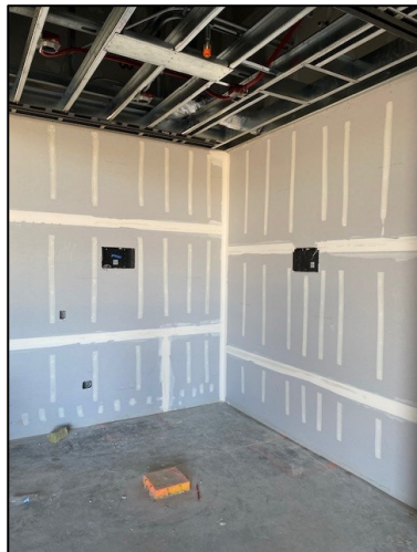
Drywall Tape – 1 st Floor
