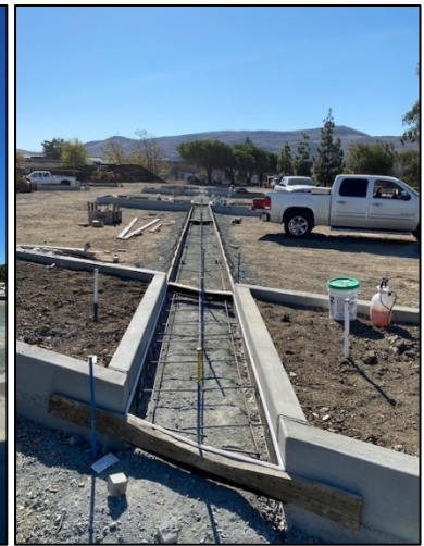
Concrete Formwork – Lot 4
