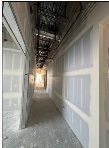
Drywall – 1 st Floor
