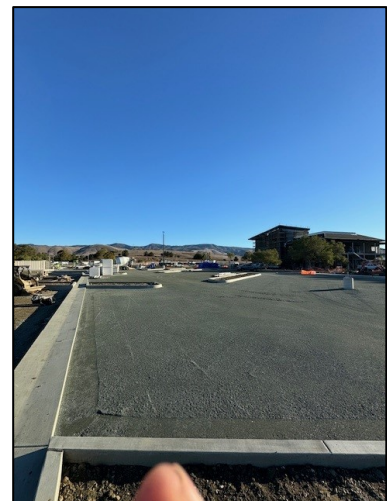
Base and Concrete – Lot 4
