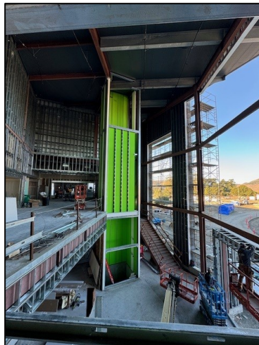
Framing at Elevator Shaft
