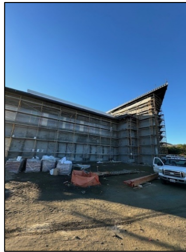
Exterior Plaster – West
