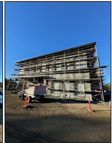
Exterior Plaster - North
