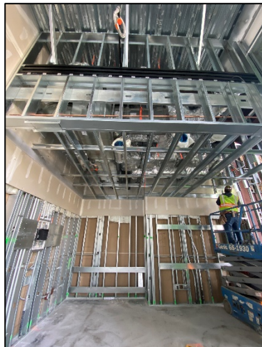
Metal Stud Framing – 2 nd Floor
