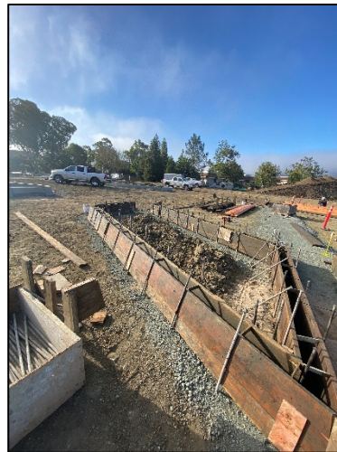
Concrete Formwork – Lot 4 Underground Electrical – Lot 4
