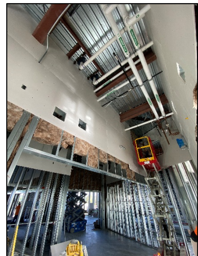
Drywall Installation – 2 nd Floor
