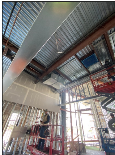
Duct Work Installation – 2 nd Floor
